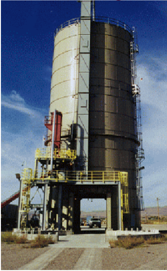
These silos are examples of field bolted tanks with truck drive through bays. Notice Height:Diameter ratio
