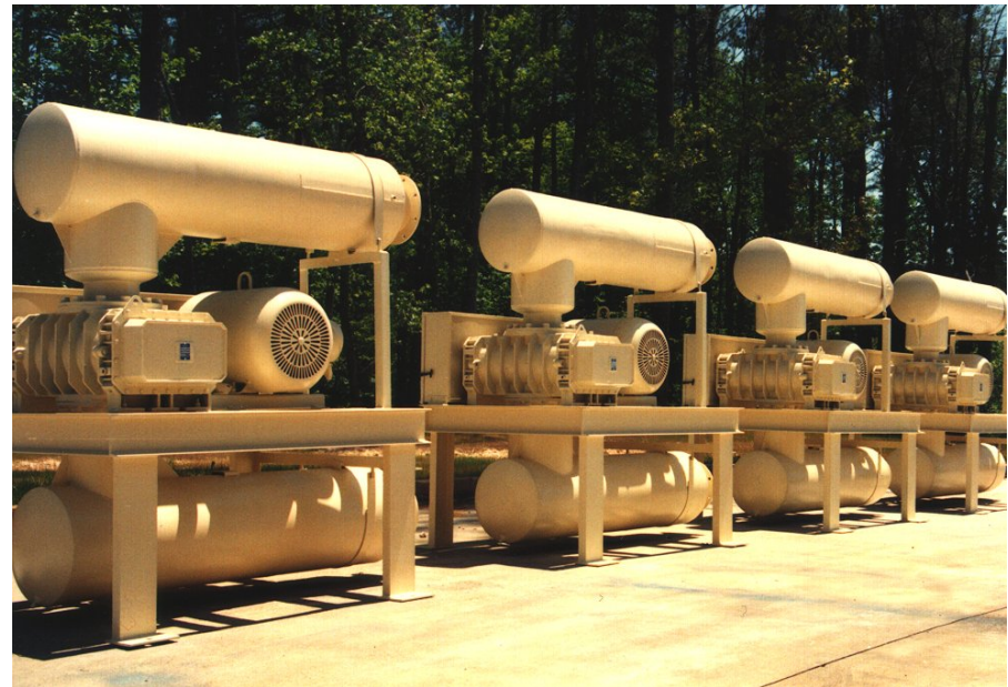
Elevated base mounted vacuum blowers
