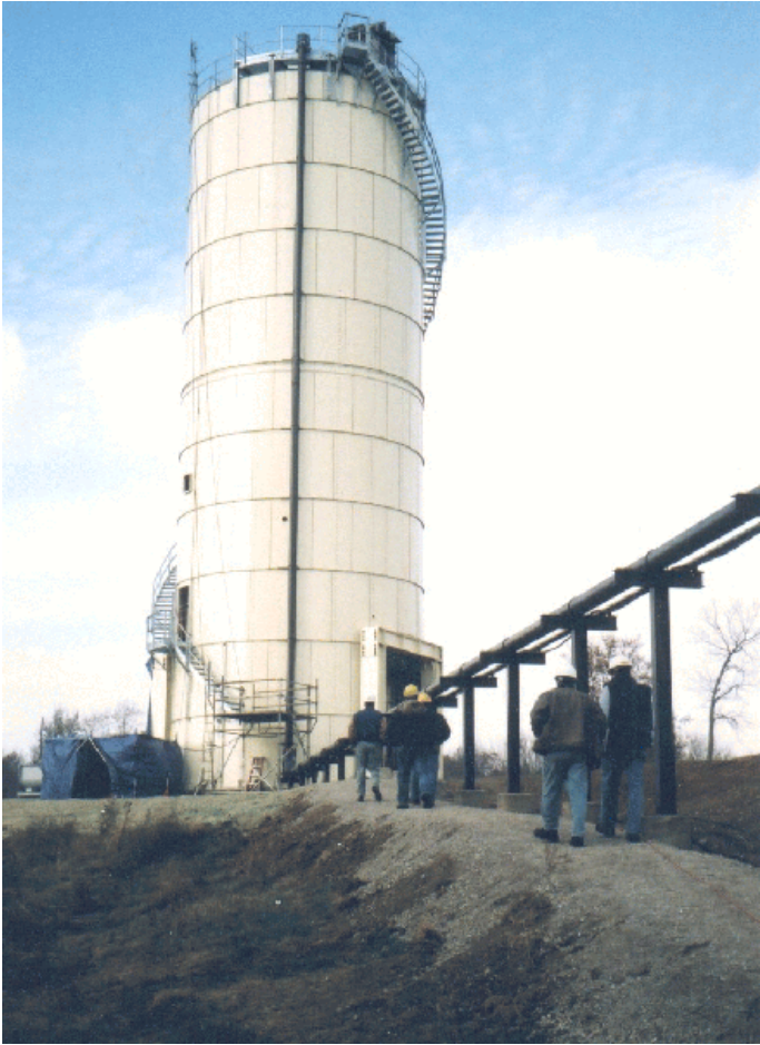
These silos are examples of field bolted tanks with truck drive through bays. Notice Height:Diameter ratio
